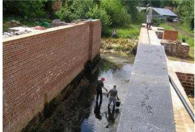
*Inside Bacton Wood Lock before the chamber was finally drained down. Already there is a steep drop down from the top sill as shown on the left, whilst on the right the volunteers clear small fish from the chamber. (Alan Bertram)*
