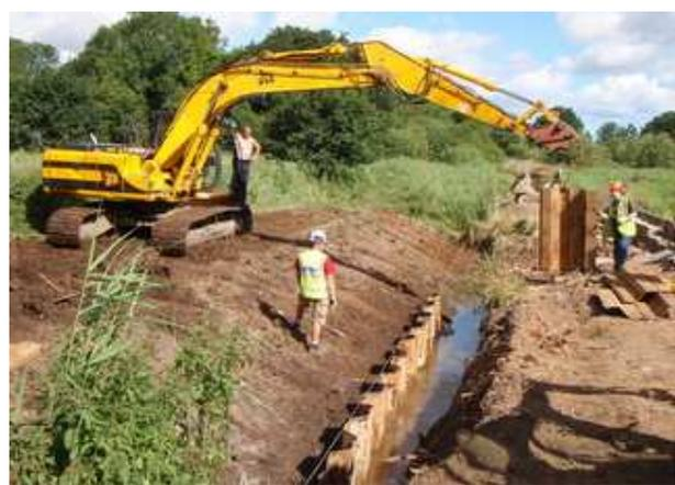
(Left) The start of the quay heading work alongside the site of the former Wherry Inn at Royston Bridge whilst (right) a short distance away work gets going on the complete rebuilding of the old spillway.
