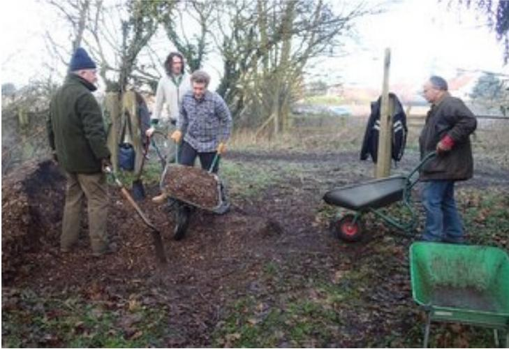
**Honing Staithe Walk:** On 12 January 2014 many barrow loads of chippings were laid on the path through the wood to consolidate the surface for walkers. When it was created the path had to be routed through low lying land that was liable to flood and building up its surface will make for a much firmer surface in future.
