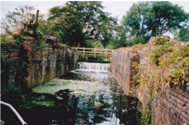
*Honing lock on 31 August 2003 after some preliminary clearance had been carried out by the working parties. The stumps of two large trees on the left were still to be dealt with. The picture was taken from the bows of a motorised work boat that had been used by a group of EAWA directors to inspect the state of the canal up to the lock and to view the progress of the lock clearance work. (Picture from the Editor's collection)*
