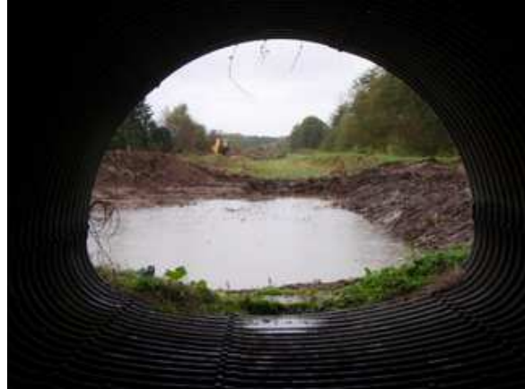
Royston Bridge : Left: Removing the stop soil to determine if the original clay lining of the canal was still intact. Right: A subsequent view through the bridge following heavy rain indicated the bed remained watertight.
