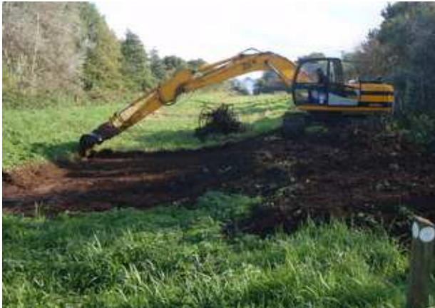
Royston Bridge : Left: Removing the stop soil to determine if the original clay lining of the canal was still intact. Right: A subsequent view through the bridge following heavy rain indicated the bed remained watertight.
