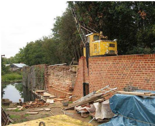
As members will know the Ashtons have made great progress in restoring Bacton Wood Lock with major assistance from our voluntary work parties. The upstream fore bay has been rebuilt, some repairs have been carried out to the chamber, and thoughts are now turning to the building and installation of lock gates.
