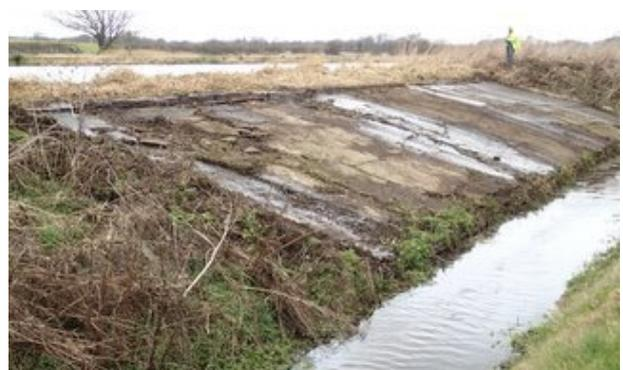
A major objective was achieved on 23 February when the overgrown spillway, above Ebridge Lock, was cleared enabling it to be able to function by allowing surplus water to flow into the back soke. Some repairs will eventually be needed but in the meantime this important flood protection measure is now fully functional.
