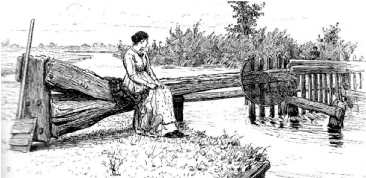
The barge could now bypass the mill, but, between mills, the rivers could still be shallow, and in many places forded by the local carts. Here, staunches would be built, perhaps only raising the water level by a couple of feet, and usually set open to allow the fords to be used, being closed only for the duration of a boat passing. For some fifty years, the staunch at Tempsford was only closed late at night so as to
