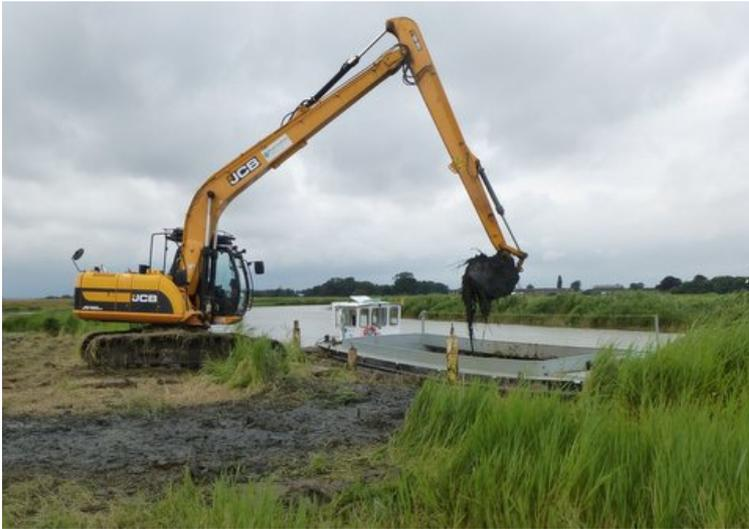
Another development is the retirement of the old steel-hulled barge with a crane mounted on it; this has been replaced by a versatile long reach excavator which will sit on linkflotes and dredge using a new hydraulic clam shell bucket. Over the last four years the Authority has purchased three of the long reach hydraulic excavators and a set of four linkflotes.
